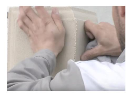
To achieve the most successful adhesion possible, the glue mixture should be applied to the entire length of the moulding and the desired application surface using a notched trowel.
