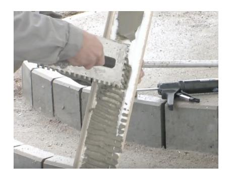
When fitting mouldings, the air temperature should be within the region of  $5\,^{\circ}\text{C}$  and  $30\,^{\circ}\text{C}.$
