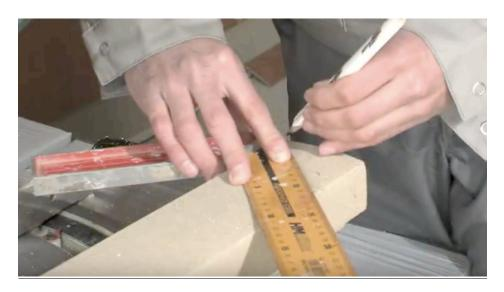
Our mouldings can be cut using most commonly used tools such as a metal hand saw, however we advise using a circular saw for cutting precise and clean angles.
