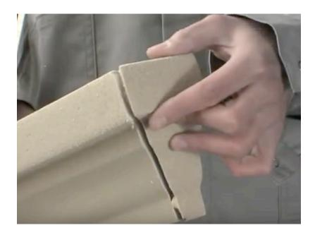
After the glue has dried the join should be filled out with extra glue and the surface smoothed to achieve a seamless finish.
